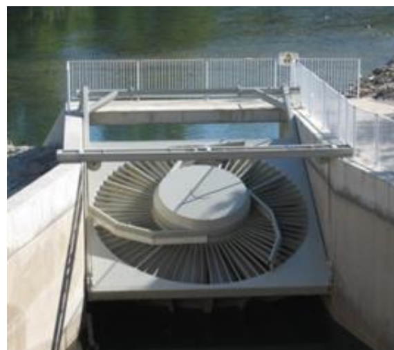
A VLH in lifted maintenance position.
