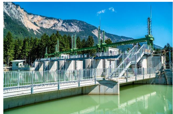
Renewal of 80 years old weirs structure and steel mechanical equipment, hpp Schütt, Austria.
