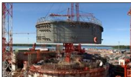
Nuclear Power Plant, Containment Liner (at that time under construction); © Babcock Noell GmbH (nowadays Bilfinger Noell).
