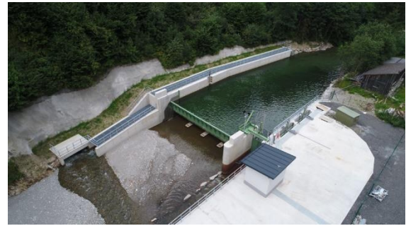
Intake with fish pass, hpp Kremsbrücke, Austria.
