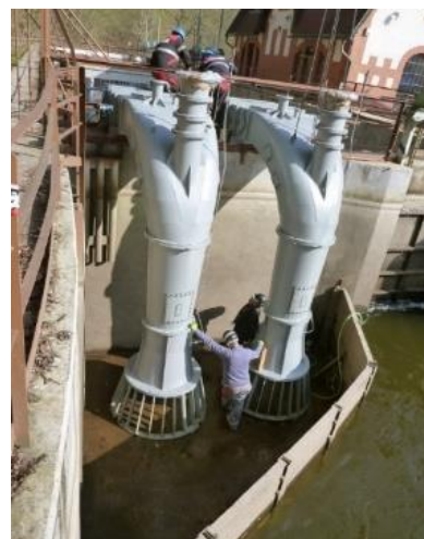
Installation of siphon low head turbine.
