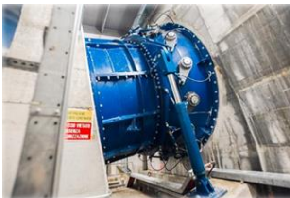
Wicket Gate mechanism for the same Turbine Runner Ø 2,800 mm 2,000 kW.
