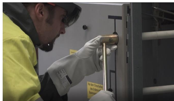
Switching operations in a medium-voltage network.
