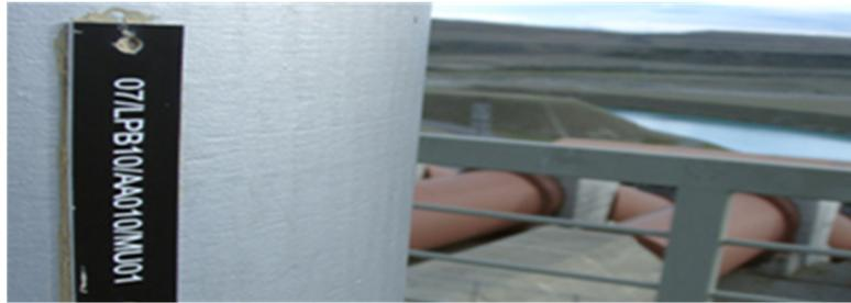
The **KKS** Power Plant Identification System was developed by planners and operators of the German power plant industry and published in 1978 as a national guideline of vgbe (former VGB Technischer Verband der Grosskraftwerksbetreiber e.V.). It has been used worldwide for decades in more than a thousand power plants and has become “acknowledged rule of technology.”
